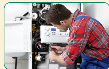
Have your heating system serviced annually
