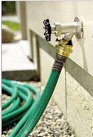
Hose bibb vacuum breakers shown left and above, are effective in preventing contamination.
