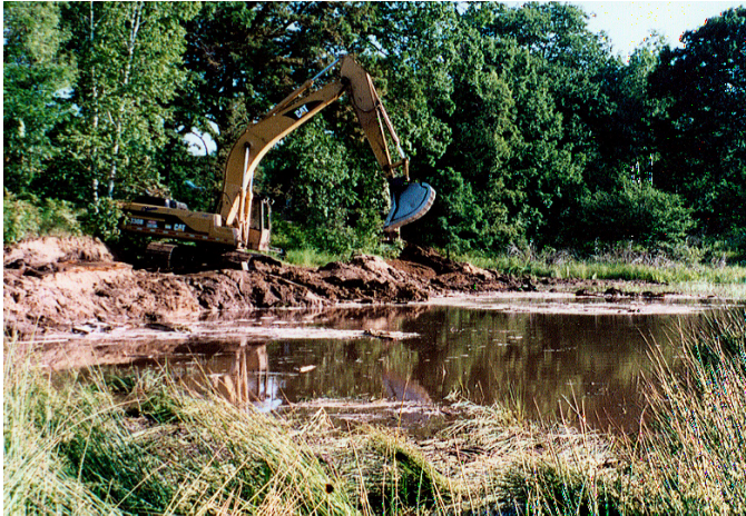
Figure 13. Drag-line (backhoe) dredging.
