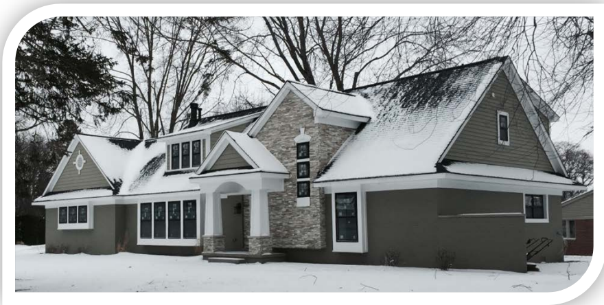
(Above picture: Second Floor Addition with façade renovation)
