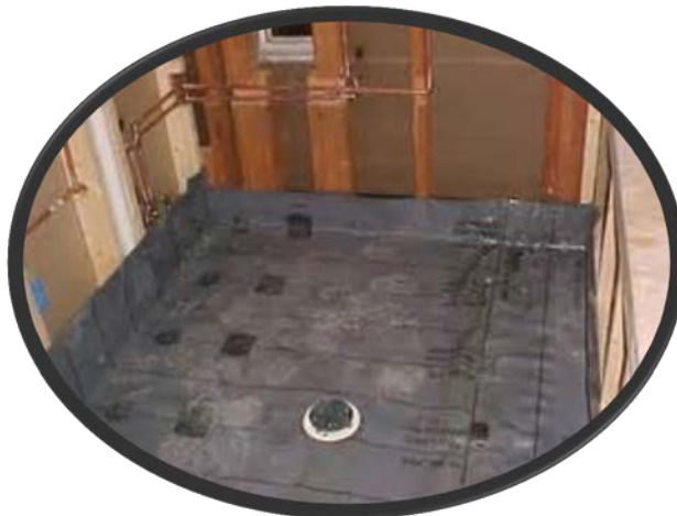
(Above picture: Installation of a shower pan)
